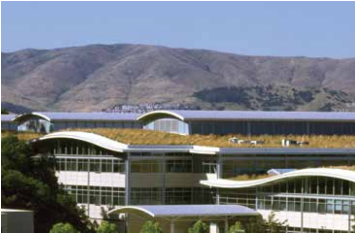
A green roof on the offices of YouTube in San Bruno, California.
